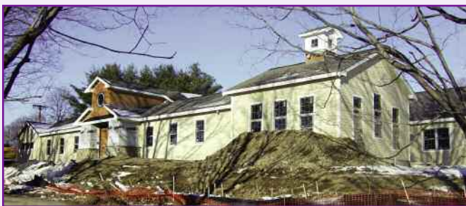
Construction nears completion at Spectrum's new Women & Children's Center in Westborough, Massachusetts.
